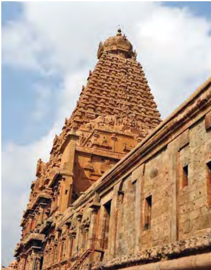
Fig. 4 | Bṛhadiśvara Temple, Main Sanctuary Tower
